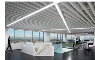
Manage and optimize lighting
