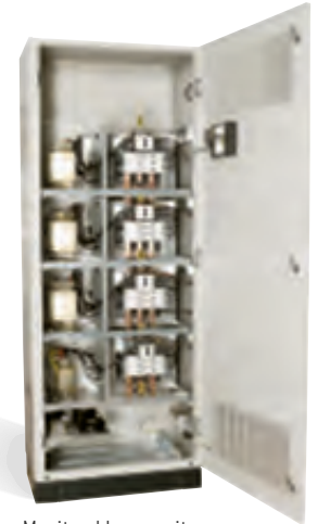
Monitorable capacitor banks improve the voltage level at the end of the line.
