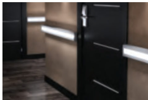
Illuminated trunking with low consumption LED lighting to guide people in passageways.
