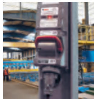
Fusible Mechanical Interlocks, extra-rugged construction, NEMA 4X and 12 watertight rated.
