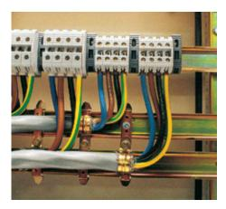
\* For a real "bonding" approach: earthing of shielding by clamps fixed on "Fixomega" claws clear identification of the circuits on Viking terminal blocks
