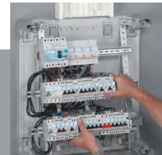
XL<sup>3</sup> 160: After complete removal of the frame and side panels, full access for wiring.
